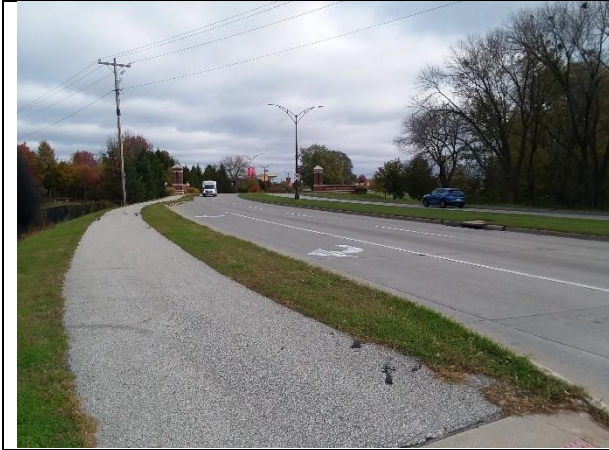
The sidepath on University Boulevard has a landscape buffer.
